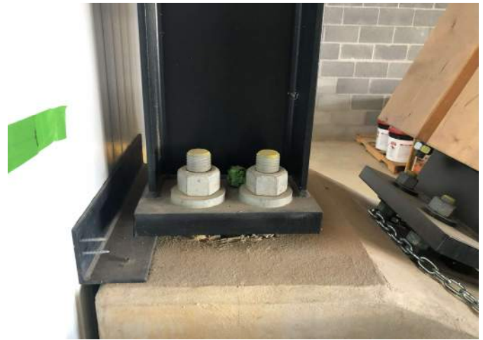
Heavy timber steel connection system.
