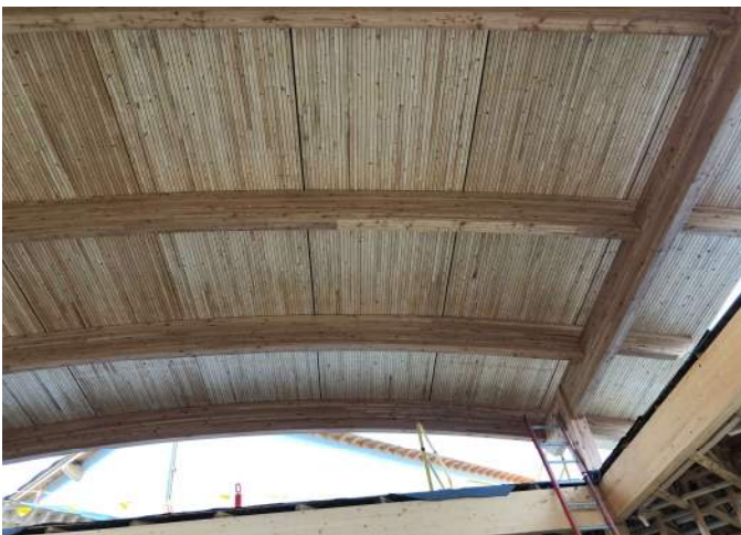
Timber system at main entrance to UMT Community Center.
