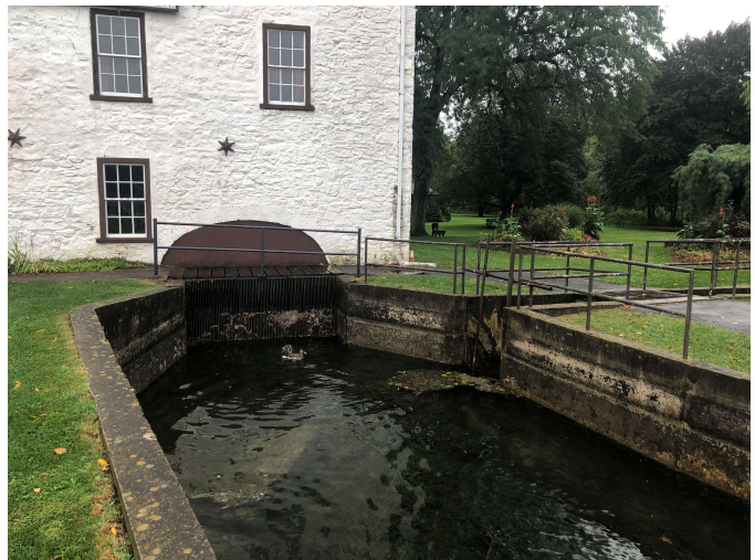
Water Flume Which Fed The Water Wheel
