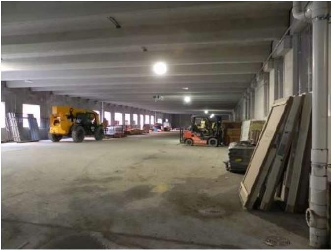
The Parking Area Is on Two Floors
