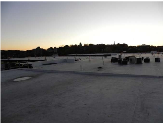
The Full Expanse of The Roof
